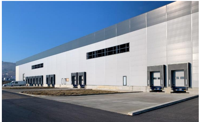
Figure 4: Zagreb Logistics Park – Hall 4
